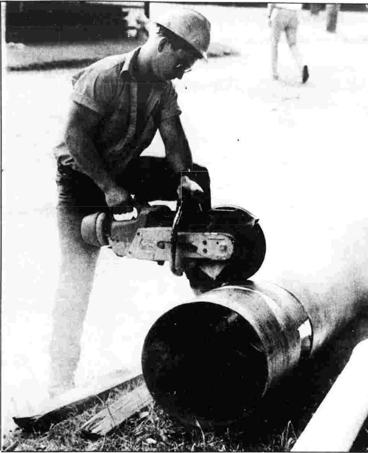
ON THE JOB — Dan Guachione of 19 Tania Drive in Manchester, uses a power saw to cut through a tube for the sewer construction on Keeney Street. Guachione works for the Glenn Construction Corp. of 86 Sanrico Drive in Manchester.
